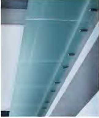
The overlooking view to the proposed terrace will be obscured by frosted glass screen
